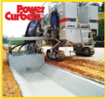
Slip-Forming Concrete Curbs & Gutters
