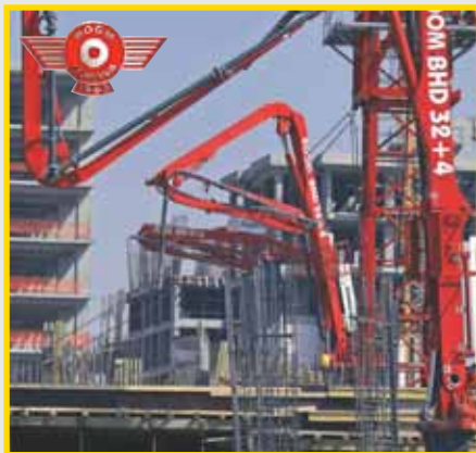
Concrete Placing Booms
