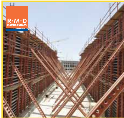
Formworks & Falsework Solutions
