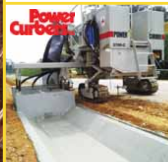
Slip-Forming Concrete Curbs & Gutters
